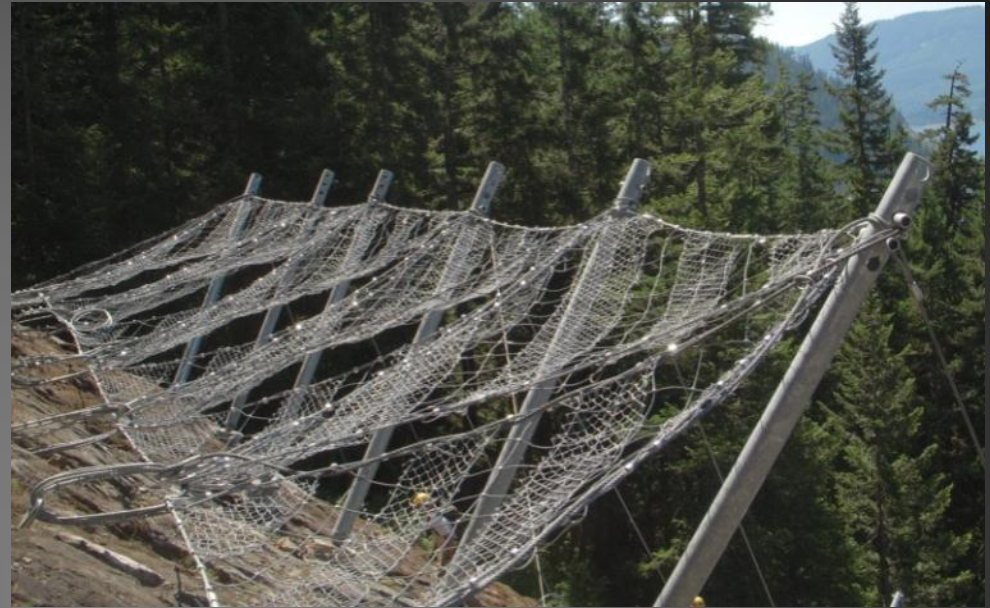
“Bald Knob” I-90 Snoqualmie Pass East Photo: Hi Tech Rockfall
