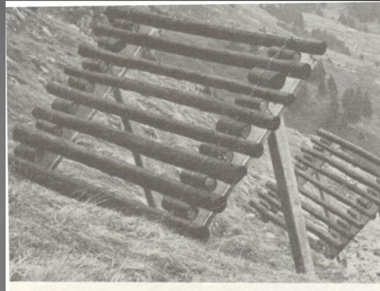
Aluminum Frame with Wood Cross Members 1959 photo by Wagner & Hopf Mattstock Avalanche Amden, Switz.
